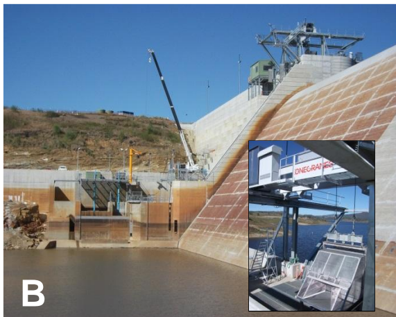
Plate 4: Photos of special lift solutions: A + B the inclined fish lift at Wyaralong dam (from: Richard Herweyten, Hydro Tasmania), as well as C + D - photos of the inclined fish funicular at Frieira dam (from: António Pinheiro, Instituto Superior Técnico - University of Lisbon).
