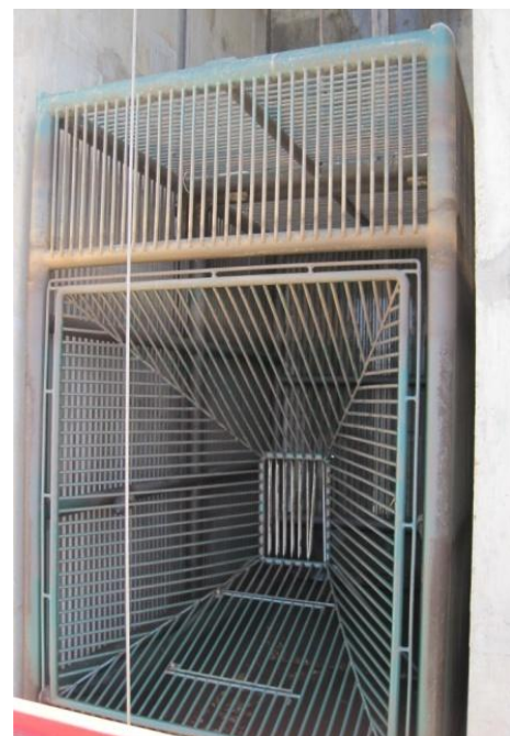
Plate 3: “Standard” construction of a fish lift, e.g. the fish lift at Grellingen in Switzerland (A) and Europe’s largest fish lift at the Pedrogão dam in Portugal (B, tower and a detail view on the fyke).
